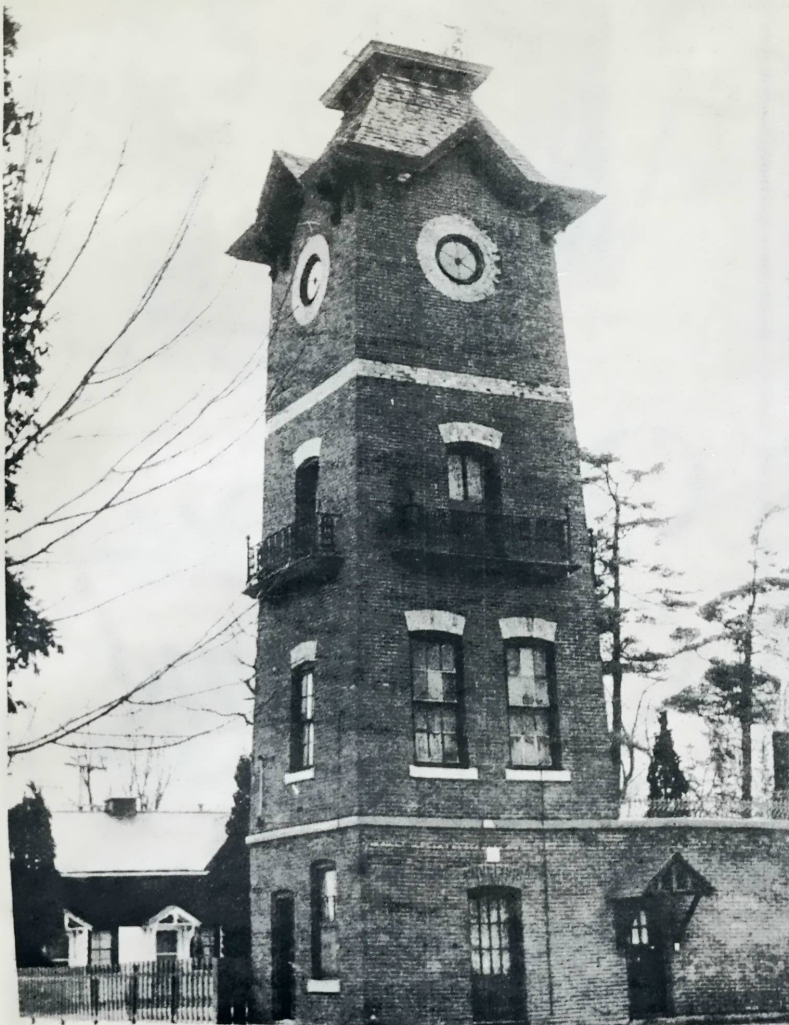
The 75 foot tower at Greenwood is of great historical significance to the community. The local Architectural Conservancy group will occupy the building starting February 7th making it their headquarters. The tower once supplied water to the home, estate and the town of Port Hope.
