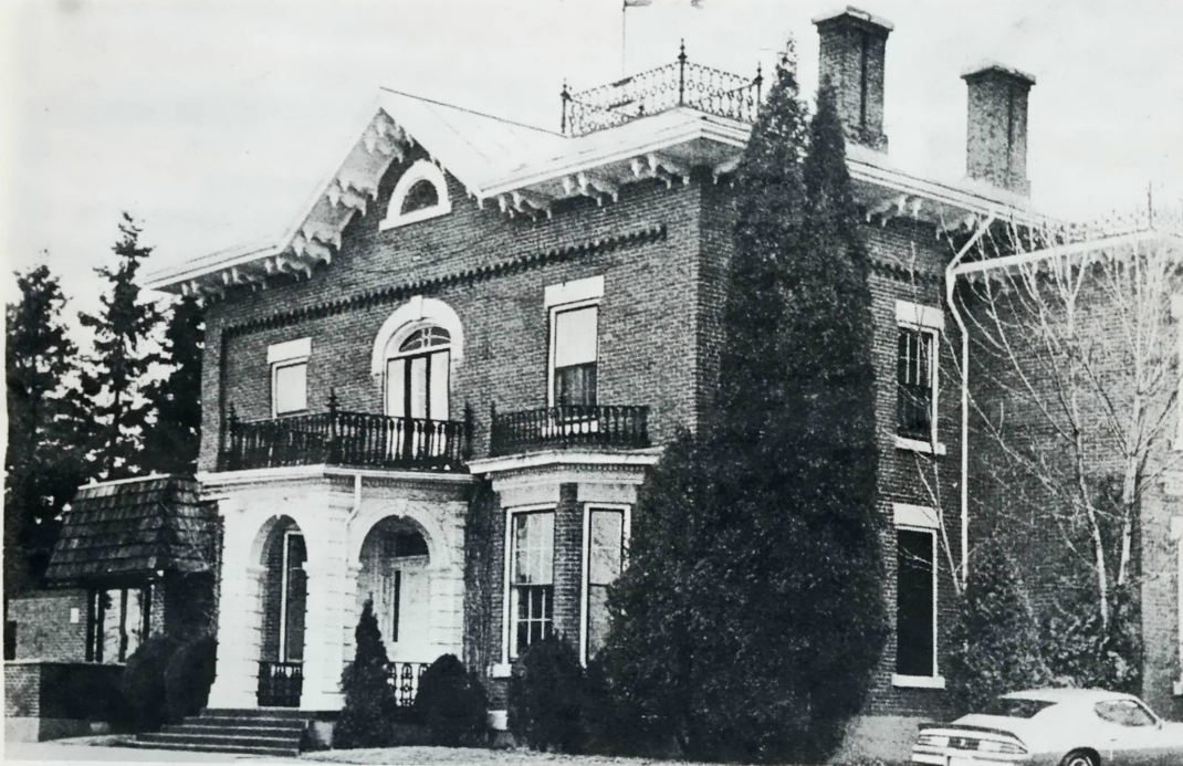
In 1866 an Englishman who owned an iron foundry in Port Hope, John Helm, set his sights on building a grand home overlooking Lake Ontario just east of the town. He arranged for the construction of what is now Greenwood Towers.
