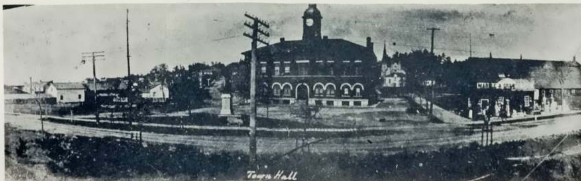
A view of the Town Hall with the Port Hope Marble and Granite Works where present day Rotary Park is located.
