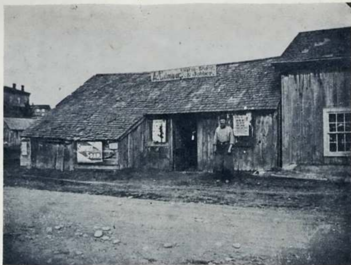
A view of A. Gilmour's Store on Ontario Street. The Robert's Store presently occupies this location.
