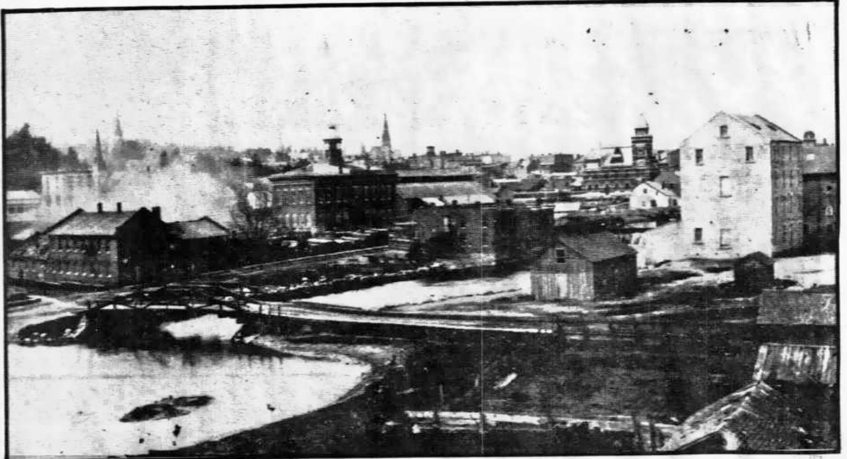
THE AGE OF MILLS — In the 19th century Port Hope was a mill town, with the southern portion of town crowded by both the mills and their outbuildings. Above, those buildings and the millponds can be seen in this shot looking north. The large building near the foreground is Dyer's Woollen Mill. (Photo from the Tom Long collection)
