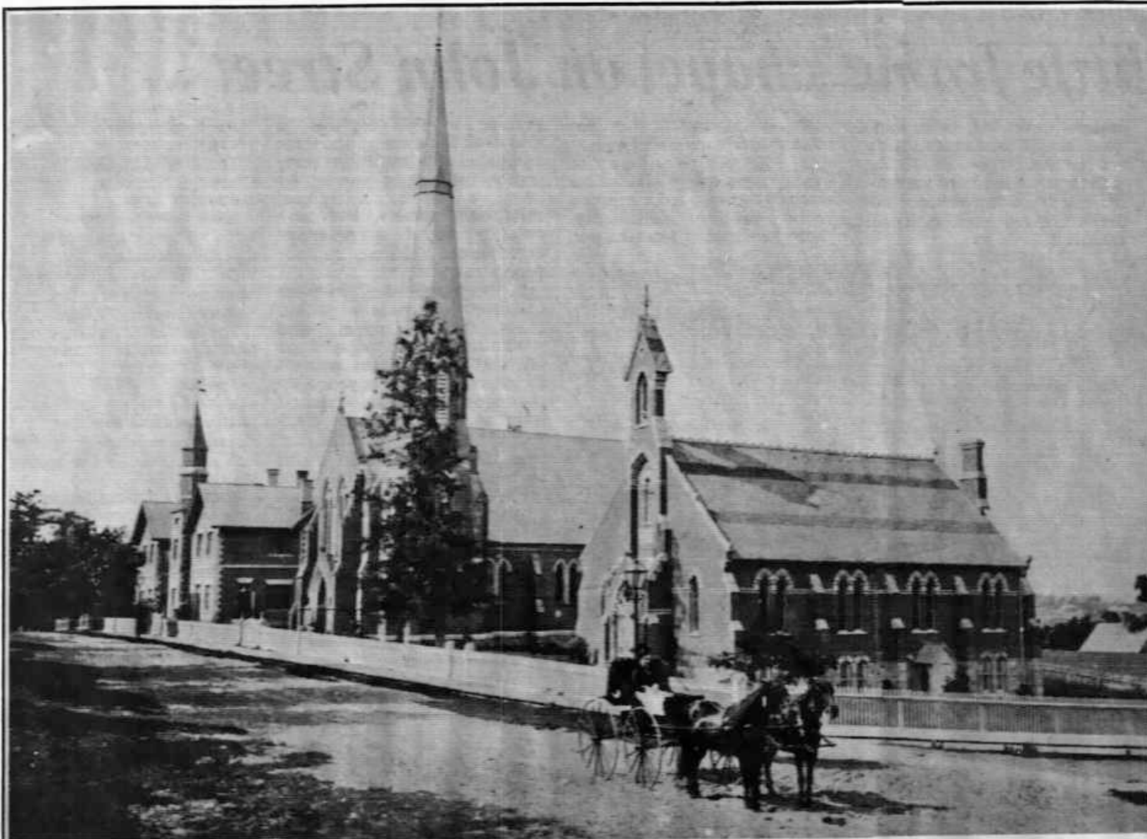
ST. JOHN'S — This photograph shows the fence which once ran around the grounds of St. John's Church — similar to St. Mark's, its parent church. St. John's was built in 1869 as a replacement for St. Mark's, because the latter was in disrepair and too small for the congregation. The parish hall, to the south of the church, was built in 1875. (Photo from the Tom Long collection)
