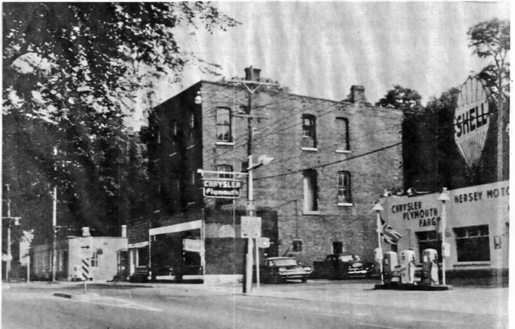
AT THE FOOT OF WALTON STREET — The large building pictured above is the first Brewer's Retail in Port Hope, used for that purpose until it was torn down in 1971. After this building was torn down, the Brewer's Retail was moved to its present location on Peter Street. Notice how different that area of town
