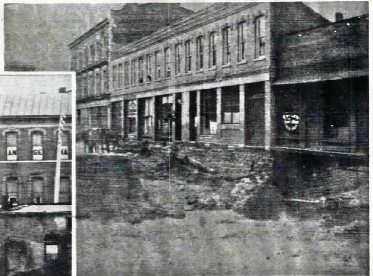
The 1890 flood washed out the Walton Street bridge (Photo from the Tom Long collection)
