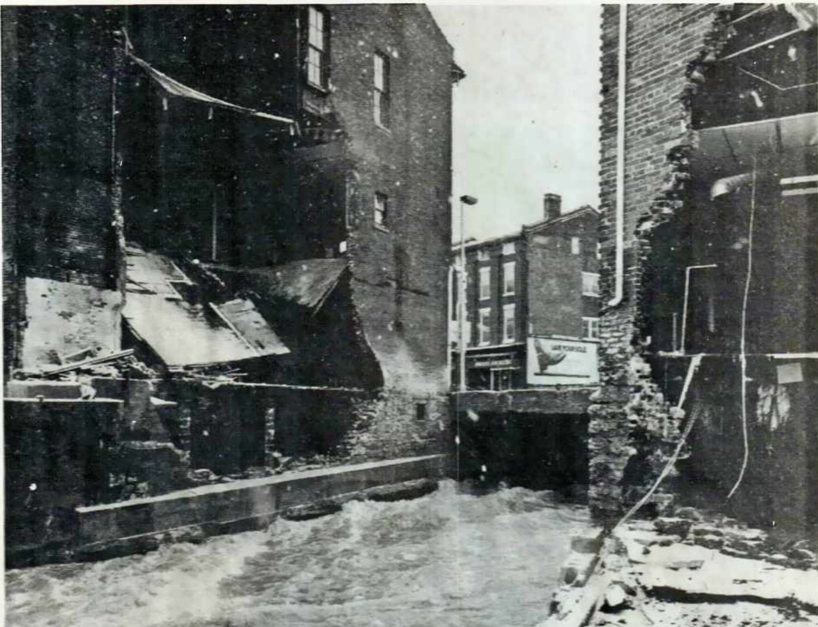
THE 1980 FLOOD — The most recent flood was also one of the most severe Port Hope has experienced. Photographs of the gaping hole which the flood left in the east wall of the old firehall (at left above) were seen in newspapers across the country; also badly damaged was Torville Terrace (the Riordan Block — at
